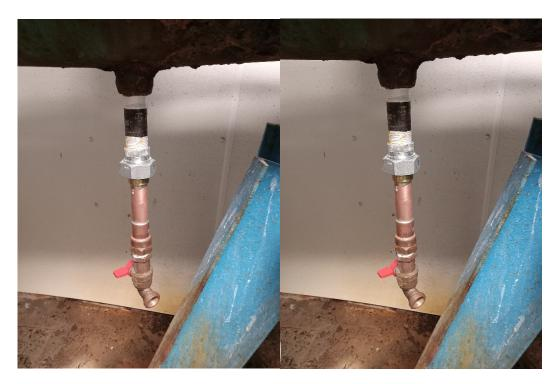
The water treatment plant needs an upgrade and repair. The corrosion from the chlorine and general atmosphere has caused the failure of the emergency repair. This would be a large project to include replacement of all the pipes exposed in the plant as well as the chlorine injection system. The failure of any part of this system will be catastrophic. We have very little components for repairing this system and our other necessary resources would be over strained to complete such a big repair.
