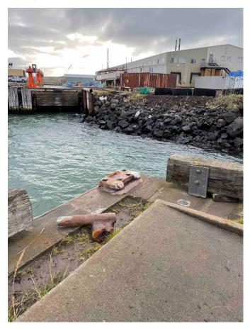
This cleat was damaged due to improper use of the winches and lack of spring line. I contacted Boyer Towing, Inc. to inform them of the broken cleat and that the City will be charging Boyer for purchase,
